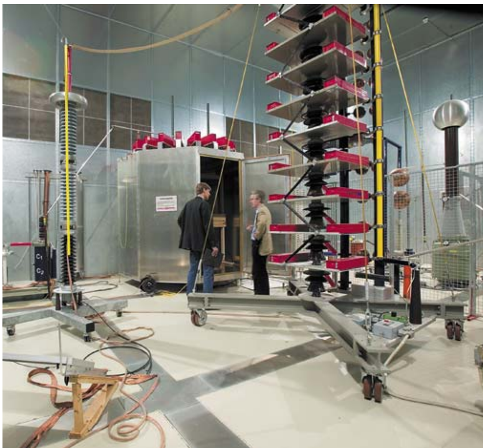
Lightning at the touch of a button: Extreme situations can be simulated in the high voltage room at the HTI PV laboratory.
